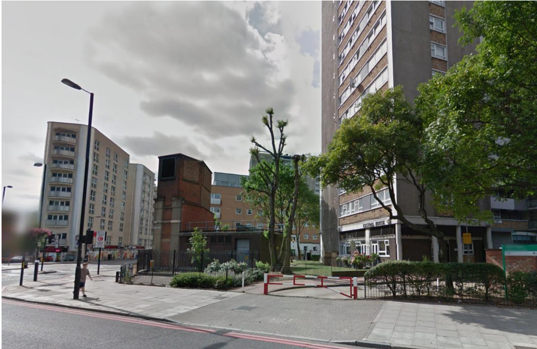
Image 4: Existing ventilation shaft building viewed from City Road looking south east towards Central Street.
