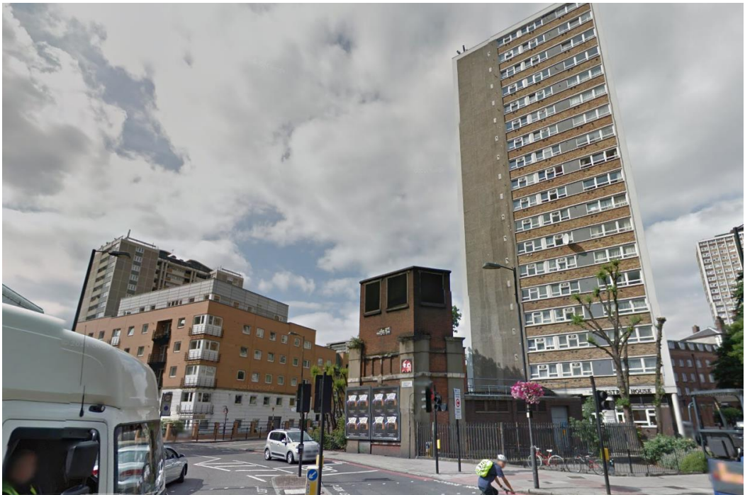
Image 3: Existing ventilation shaft building viewed from City Road looking south west.
